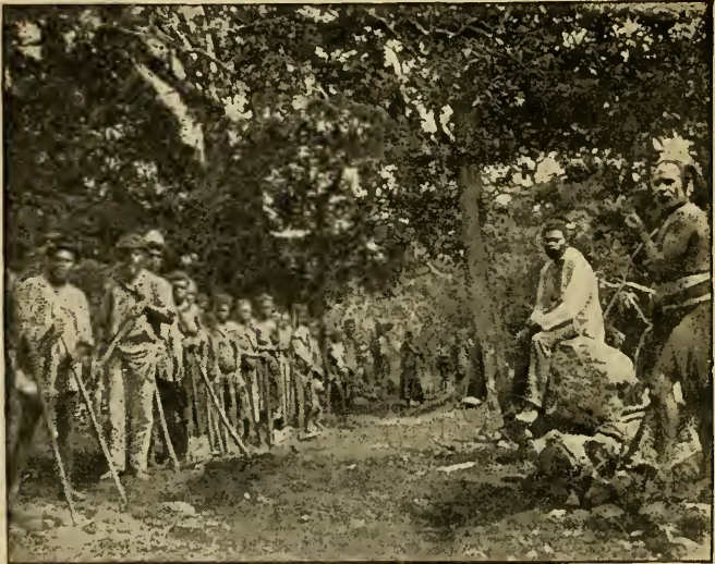
ROAD-MAKING ON TONGOA.
